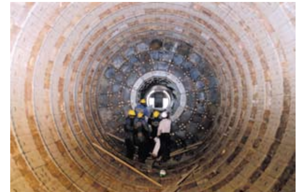
Figure 3.e Inside of a new dry kiln [57]
